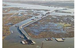
construction of a storm surge barrier and permanent closure of the Outlet to maritime shipping in April 2009. The photo shows the surge barrier under construction. The GIWW is in the foreground, the MRGO in the background.
